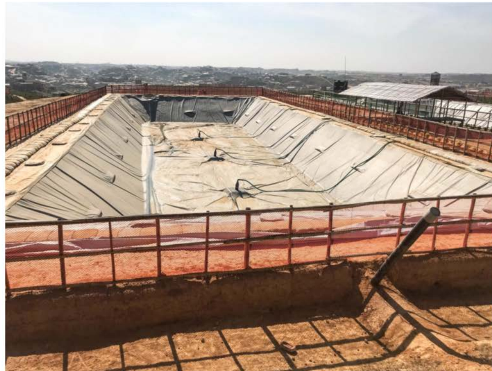
The human waste treatment facility under construction at the refugee settlement near Kutupalong, Bangladesh. © UNHCR/Firas Al-Khateeb
